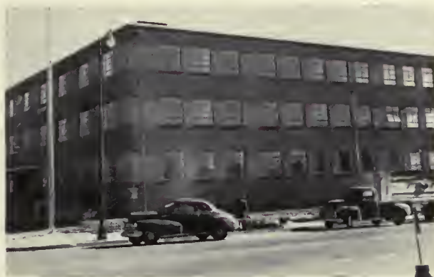
FINISHING TOUCHES and cleanup work just before the Columbia River District employees moved into their new headquarters at Ephrata, Wash. The flagpole at left had yet to participate in a flag-raising ceremony. Photo by Ellis Sharthill, laboratory technician, Columbia River District Office.
